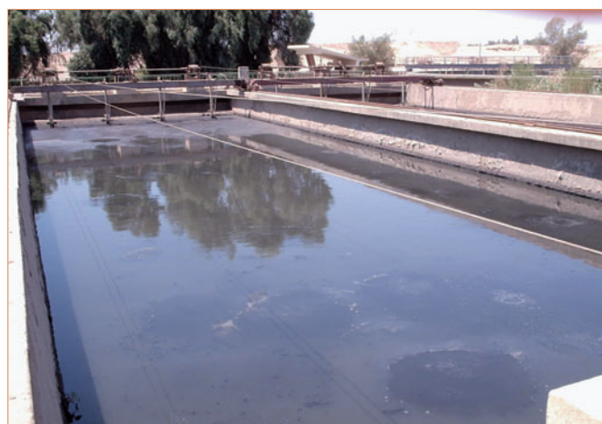
Sanitation Project Oxidation Pond, Kom El Dabai
