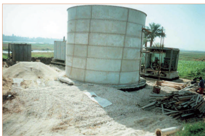
Compact Unit under construction, Naqadah
