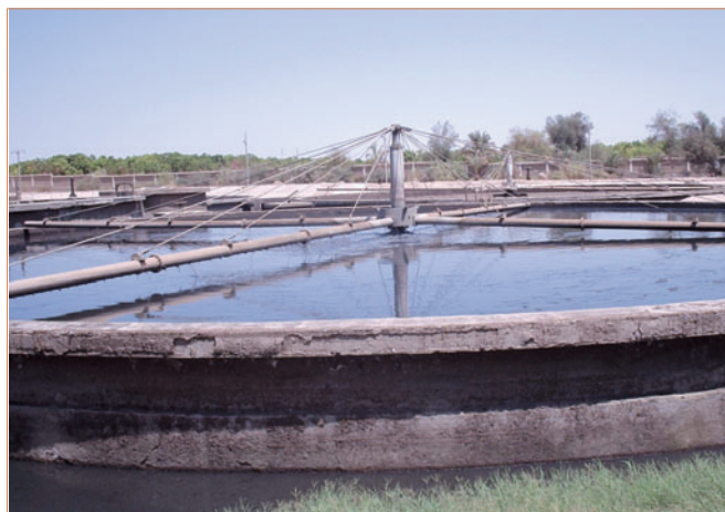
Waste Water Treatment Plant, Saleheia
