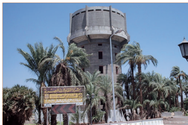
High Water Tank under construction, Qena City
