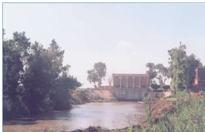
Upper Serw Pump Station
