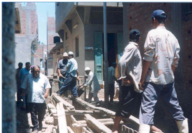
Extension of Sewer Network, Khayata Village
