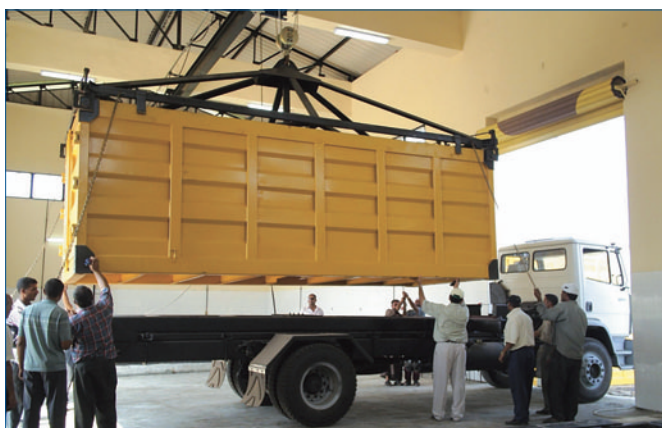
Faraskour Transfer Station
