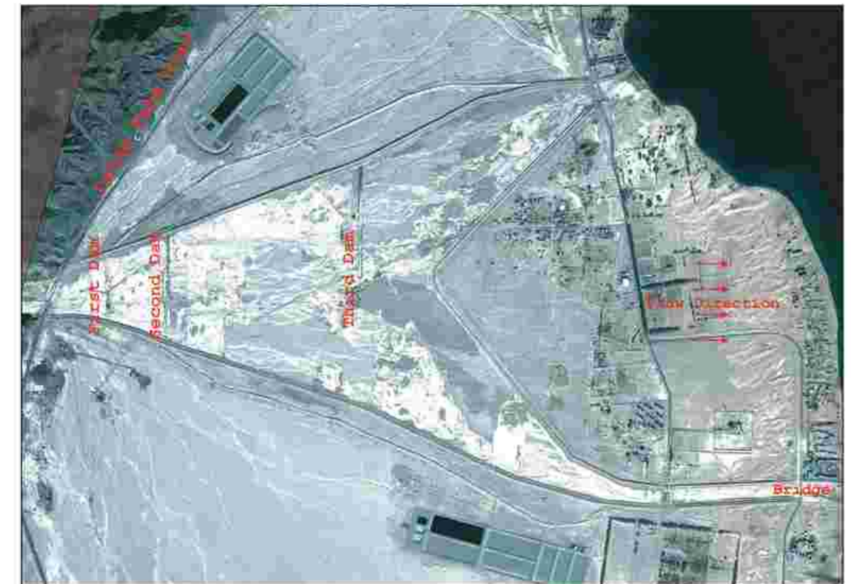
Nuweiba Flood Protection Scheme
