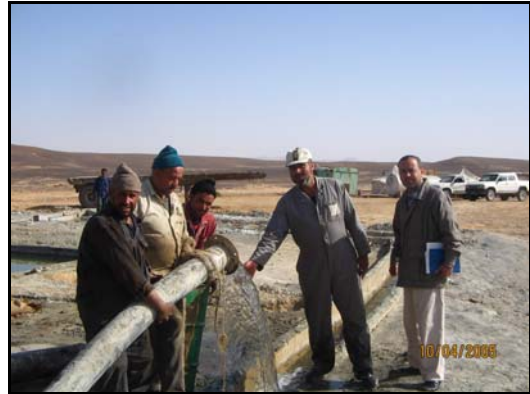
Figure (15) A groundwater well in middle of governorate
