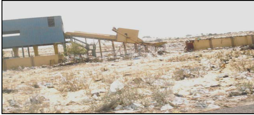
Figure (24) Arish waste recycling factory
