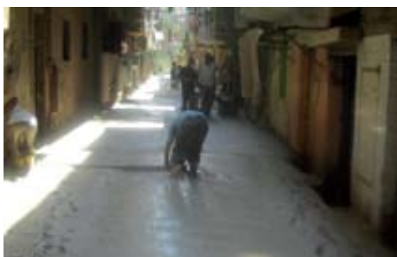
Pic. (9-6) Paving and Constructing Roads
