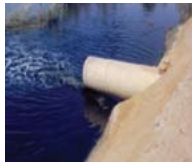
Pic. (5-7) Industrial Wastewater
