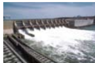
Pic. (5-5) Use of Water in Electricity Generation
