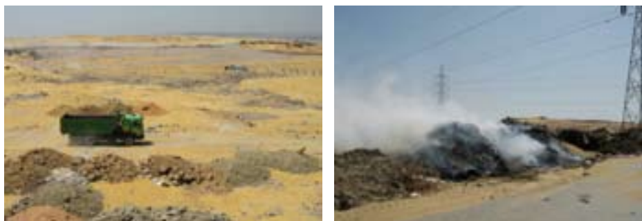
Fig (12-1), (12-2): leveling and covering Al-Wafaa & Al-Amal landfill
